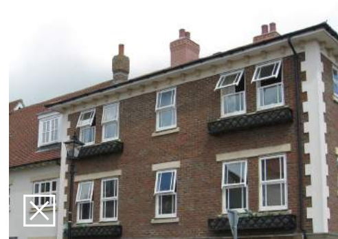
The classical styling is revealed as an unconvincing pastiche by top hung windows pretending to be sash windows
