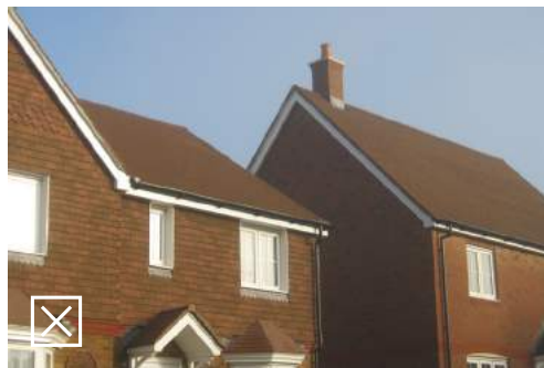
Fake chimneys should normally be avoided as they often look unconvincing and undermine architectural integrity
