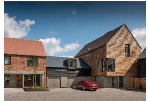
Clay hung tiles as well as brick can be effectively employed in a contemporary design. This design evokes the informal grouping of buildings and materials that might be found in a farmstead
