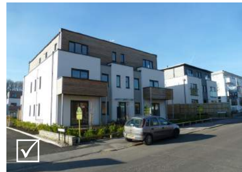
New residential development replacing employment uses on Victoria Road, Burgess Hill. establishes a consistent scale and massing and building frontage line
