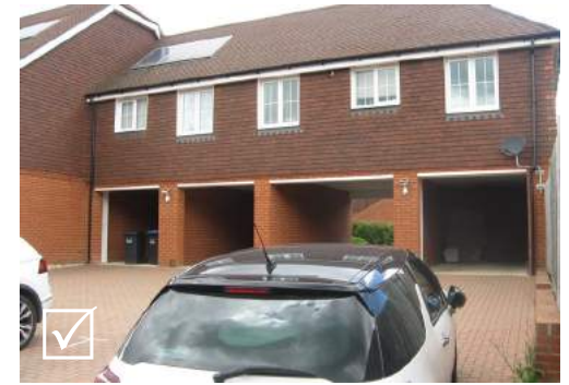
At the rear, the FOG provides direct natural surveillance over the parking court
