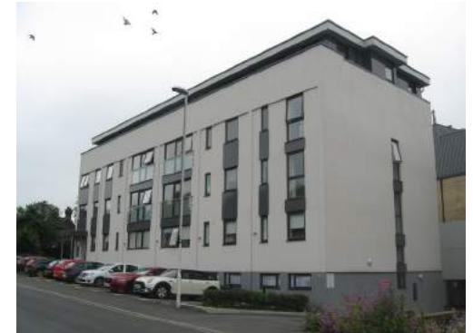
Office building in East Grinstead AFTER conversion. Whilst there are still some issues with the public realm treatment the scheme is generally a positive improvement
