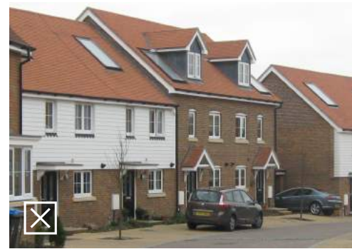
If dormers are too big this can result in a top-heavy appearance
