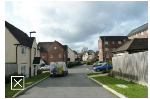
The use of close panel timber fencing to define the highway boundary is unacceptable
