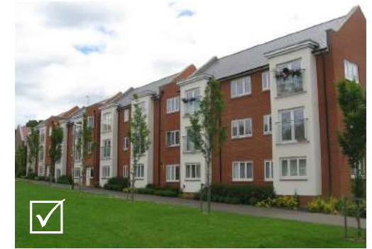
These blocks of flats have been designed so they read as subdivided facades that evoke the repeated rhythm of a run of terraced houses and sit more comfortably adjacent to smaller buildings
