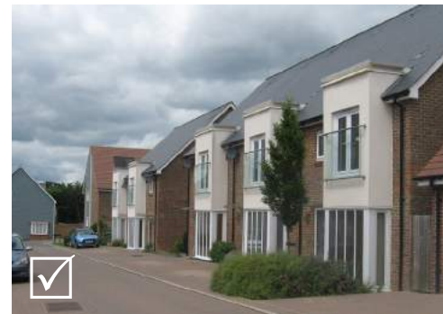
Vertically grouped windows provide elevational interest and help subdivide a frontage giving a strong rhythm when applied to a terrace of identical houses
