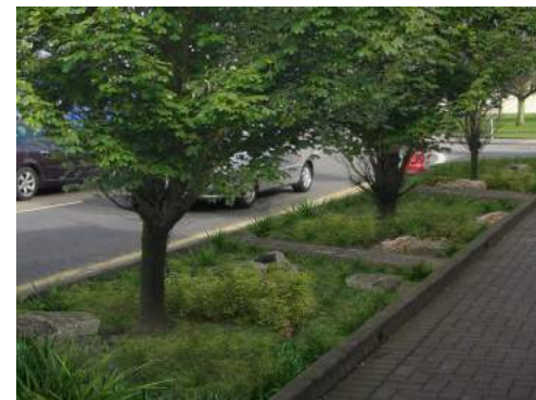
Storm water planters can be incorporated within the street design to attenuate rainwater
