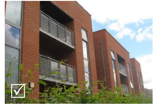
Recessed balconies integrated into design of building facade
