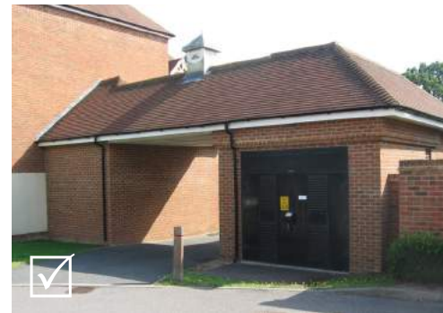
Locating sub-stations within areas of open space will not be acceptable
