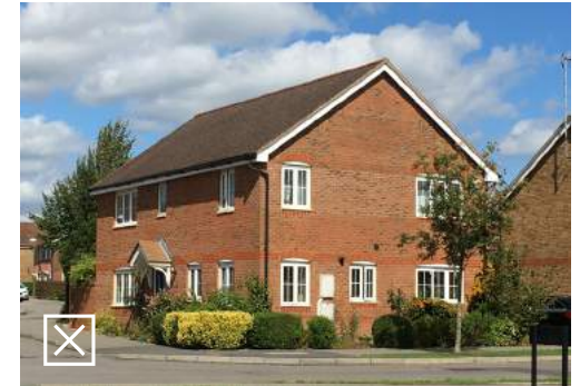
The lack of window articulation and absence of secondary facing material result in a bland façade. The elevations also suffers from inconsistently proportioned windows which incorporate fake glazing bars that undermine their authenticity
