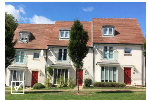
Windows have been carefully organised in a logical hierarchy that graduate in size from the ground floor to the top floor
