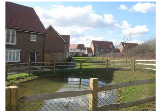
An appropriately domestic scaled attenuation pond
