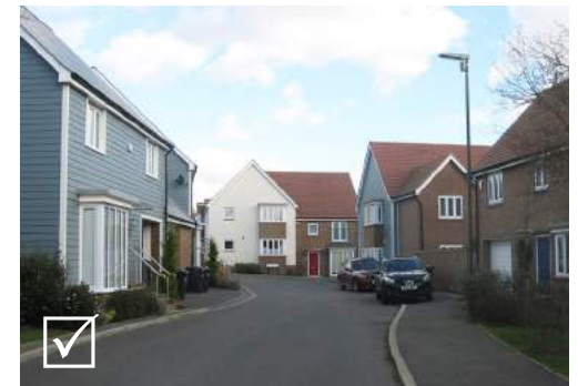
The gable flank return at the end of the street a fully fenestrated façade that addresses the end of the axis and along with the houses on each side, overlooks and animates the street
