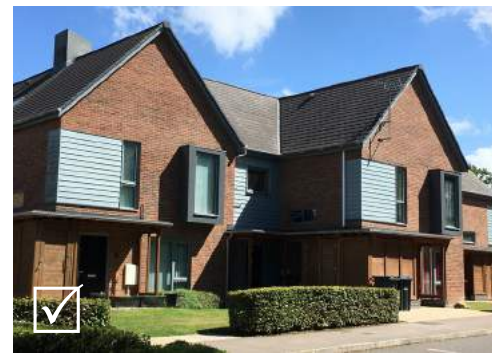
Contemporary design typically incorporates large windows and greater variety of fenestration, which may be inappropriate in a more traditional design
