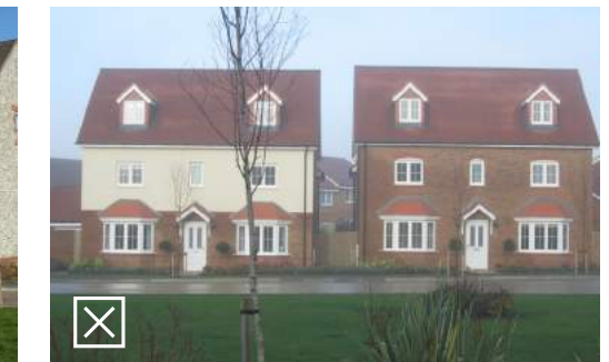
Different facing materials on the same standard building type undermines architectural integrity
