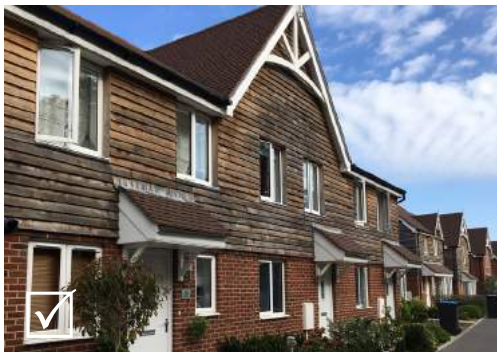
Sweet chestnut clad facades; care needs to be taken with the construction detailing to avoid irregular weathering
