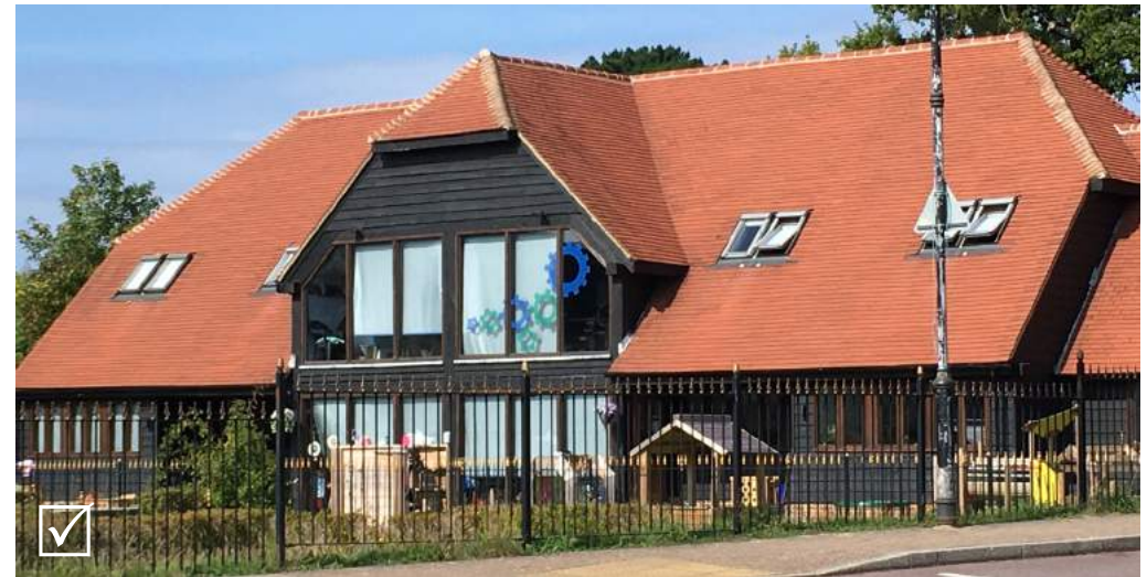
The sales office for the original Bolnore Village development has been adapted to become a children's nursery
