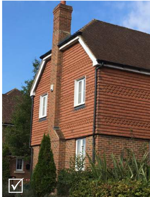
Natural clay hung (incorporating a beaver-tail pattern) tiles with local stock bricks and darker clay tiles employed on the roof
