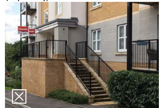
Elevating the entrance has divorced it from its street threshold and there appears to be no consideration for disability access
