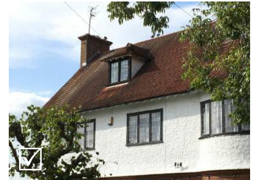
Dormers successfully integrated into the roof to provide additional space
