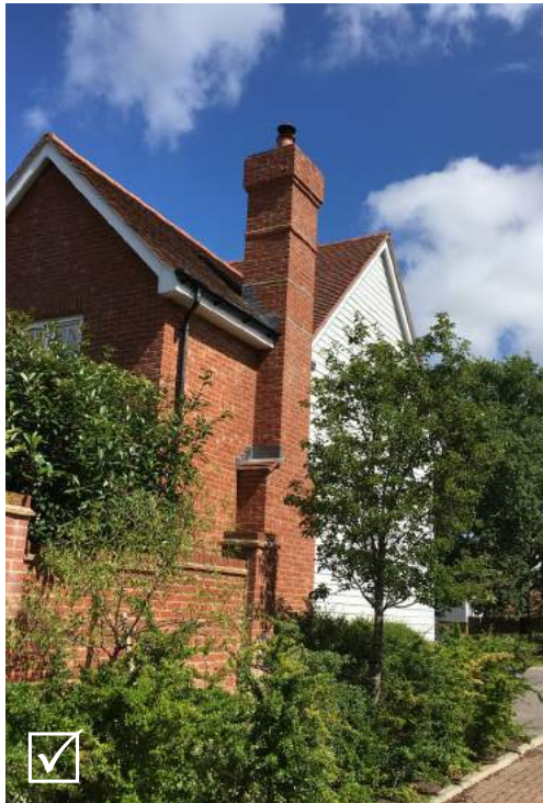
Rear boundaries facing the public realm need to be a secure height to safeguard the garden and attractively designed typically employing a brick wall and planting
