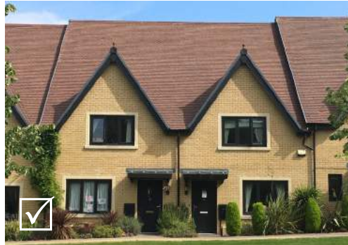
Buff brick is not typical in Mid Sussex; it has been accepted here as it echoes the colour of the adjacent sandstone-faced St Margaret's Convent and combines well with the (reconstituted) stone-framed / grey-painted windows
