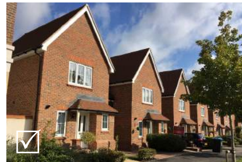
Gable fronted roofs work more successfully for narrow fronted properties
