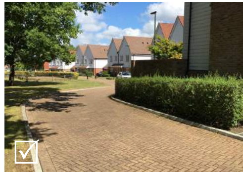
Shared surface areas surfaced in clay pavers at Imberhorne Lane, East Grinstead
