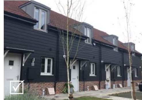
Dormer windows that extend across the eaves generate additional rainwater downpipes which if integrated in the design can work harmoniously with the façade
