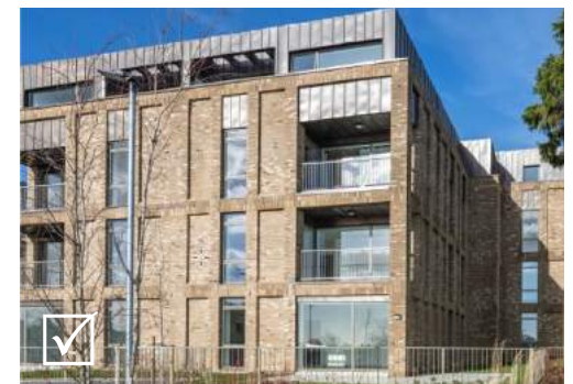
The elevations benefit from deep window reveals that add interest through the play of light and shade
