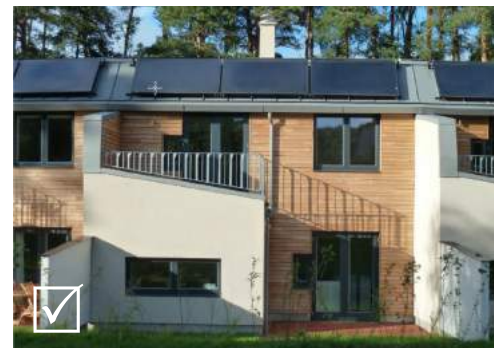
Solar panels carefully integrated into the design of a south-facing roof
