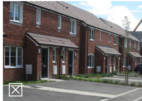
Meter boxes are prominent on building frontages
