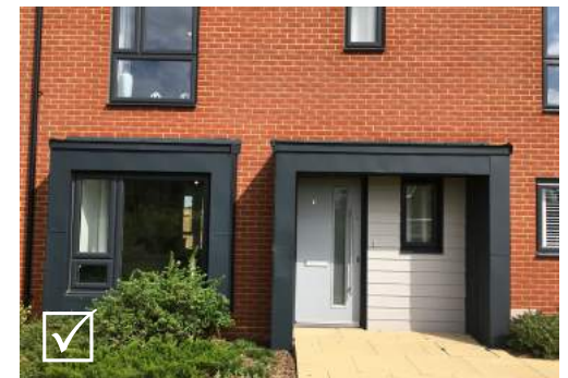
Entrances which are well defined by their canopies serving an apartment block and house (respectively)
