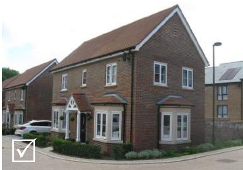
These houses address the corner well by organising the windows (and other features) so they formally address both return facades
