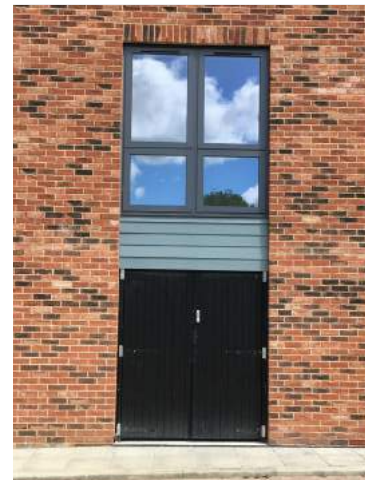
A bin store discretely accommodated within the façade
