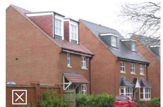
The dormers in the foreground were added and are too big and top heavy; the dormers in the background are by contrast appropriately sized
