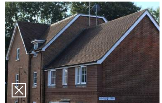
Crown topped roofs should be avoided particularly where they are visible from the street
