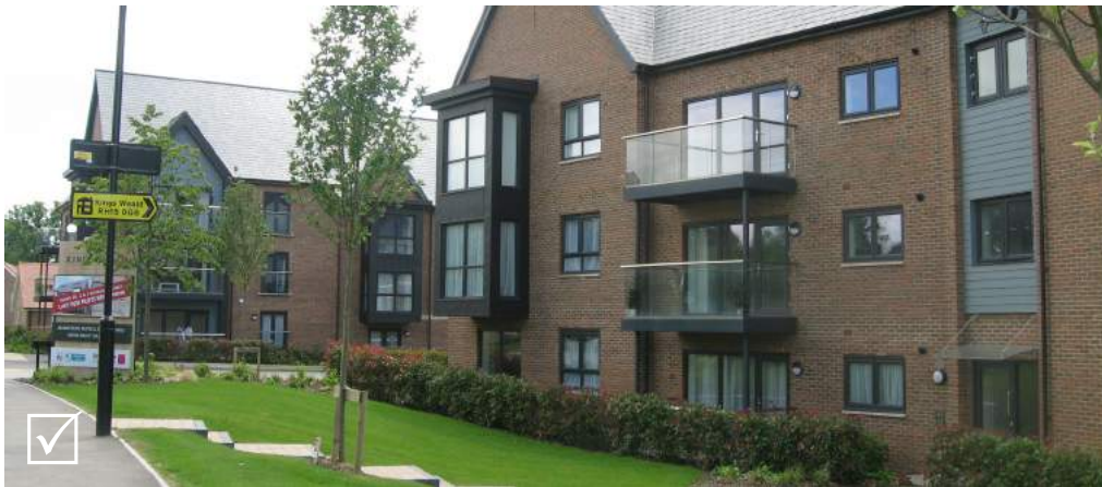
The privacy of the ground floor flats is aided by a generous planted boundary that defines the private realm while also facilitating an outlook across the public realm
