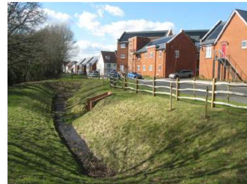
SuDs feature at Maltings Park, Burgess Hill
