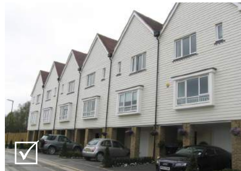
Weatherboarding can be applied successfully on a more contemporary façade
