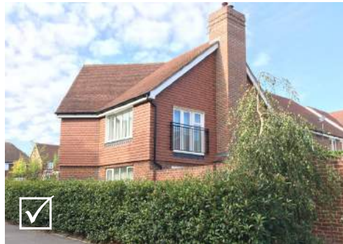
A functional chimney that is convincingly integrated into the building design
