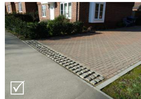
A granite sett rumble strip marks the junction between secondary and minor streets
