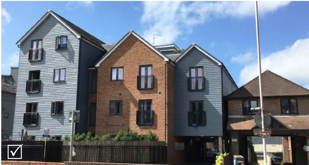
This block has been sensitively designed to step down in height adjacent to an existing lower building
