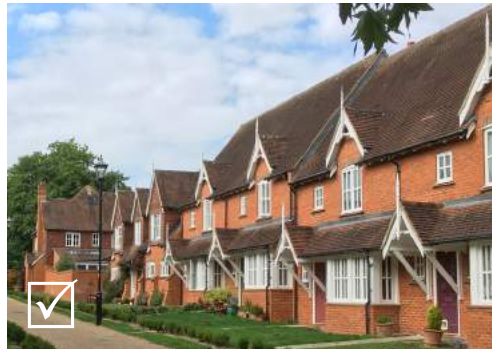
Dormer windows that extend across the eaves generate additional rainwater downpipes which if integrated in the design can work harmoniously with the façade
