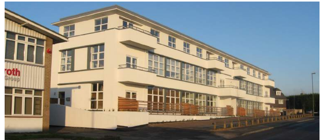
A sensitive residential conversion of an Art Deco style commercial building incorporating an additional storey
