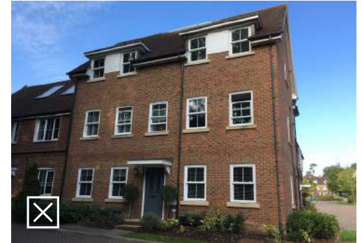
If not planned for rainwater downpipes can disrupt an elevation especially if it is otherwise symmetrically organised
