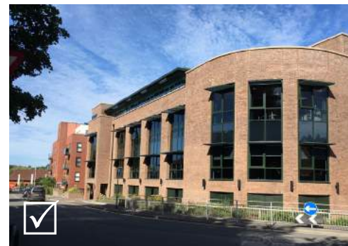
The curved corner has been designed to respond to the turn in the road and the step-up in height provides additional punctuation
