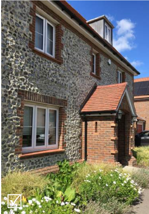
Flint facing combines well with brick detailing
