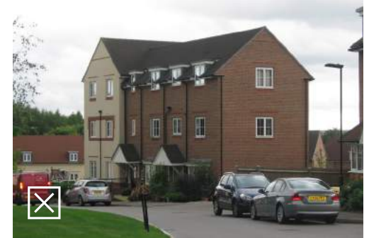
Little thought has been given to the positioning of rain water pipes, which is especially an issue when the eaves line is broken
