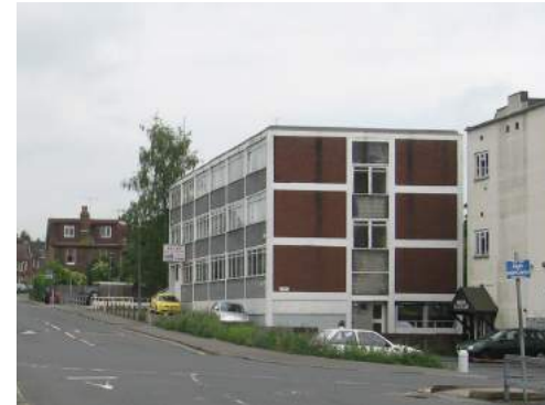
Office building in East Grinstead BEFORE conversion
